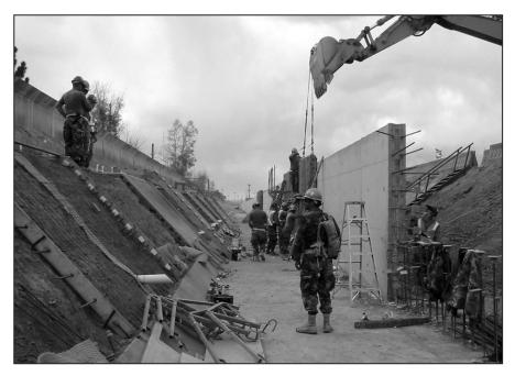
In support of the Border Patrol, U.S. Navy Seabees from Naval Mobile Construction Battalion (NMCB) 133 and NMCB 14 in March 2009 constructed a 10-foot-high wall and concrete drainage ditch along the U.S.-Mexico border at Douglas, Arizona. Photo by Petty Officer-1 Matthew Tyson.
